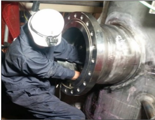
Water Jet Cut of Denitration Mineralization Reformer, Fabricated Manway and Installed
