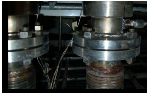
One of six Glovebox Penetration Plates to be replaced
