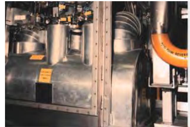
One of two existing TCAP Columns to be replaced
