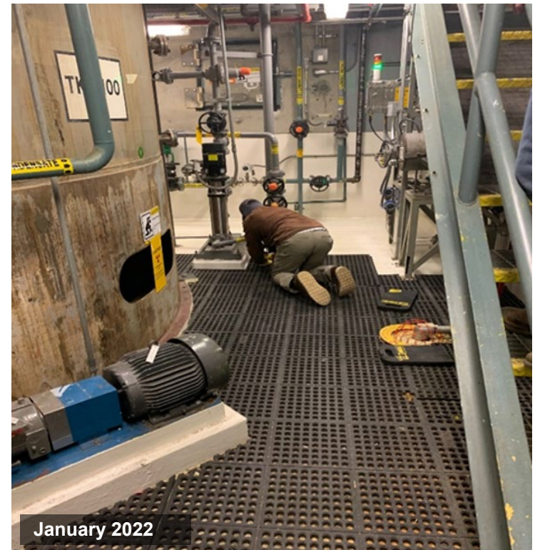
Crews removing matting in basement of 242-A Evaporator
