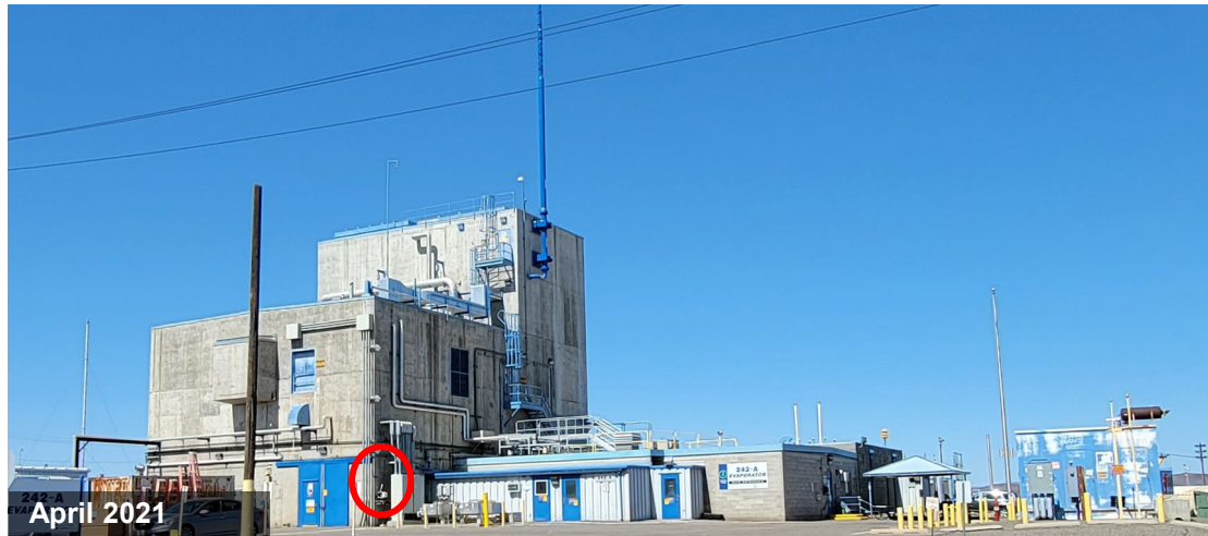
Shutdown hand switch located outside of the 242-A Evaporator
