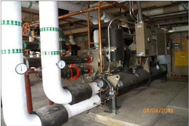
LLNL B131 Chiller Replacement
