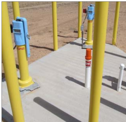
Pantex Bay/Cell and Lead In/Flame Detection System
