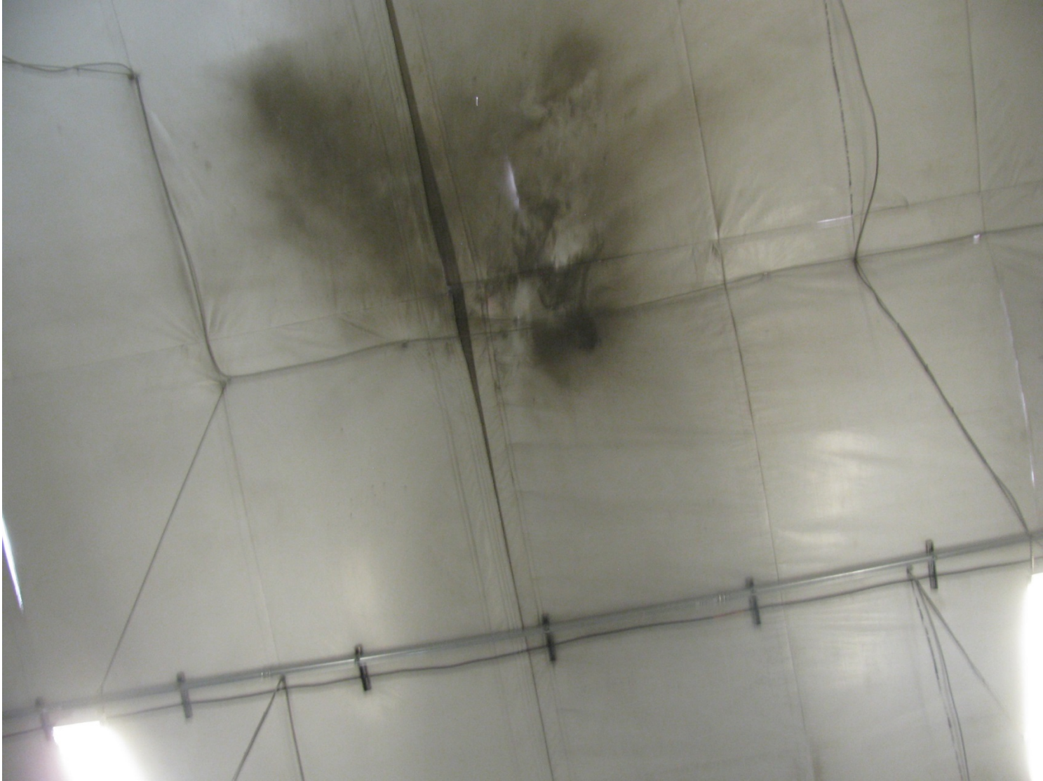
Figure 10. ARP V ceiling.
