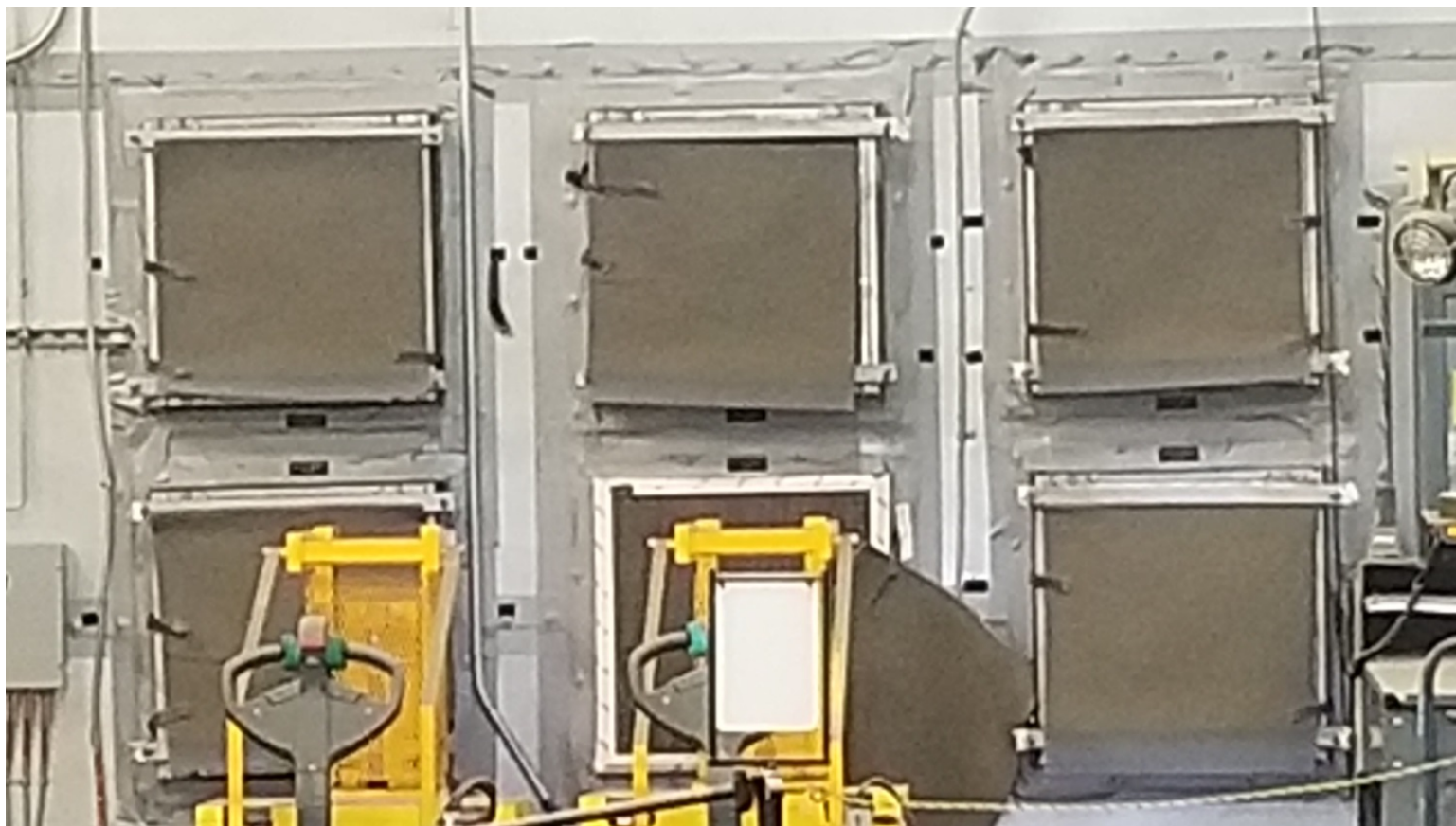
Figure 17. Ventilation pre-filters.
