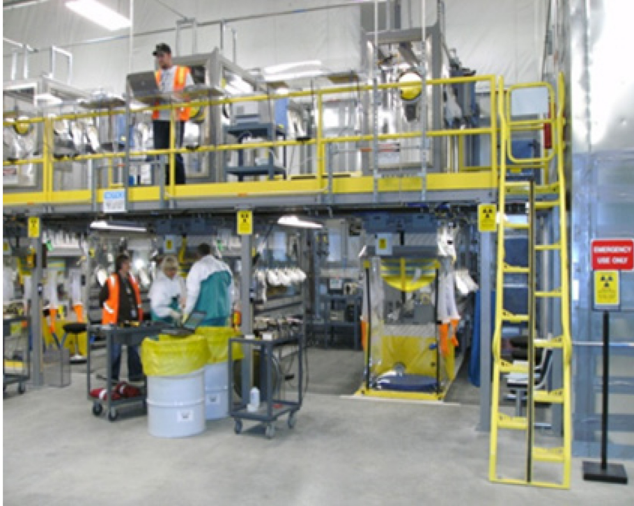
Figure 6. Drum packaging station.
