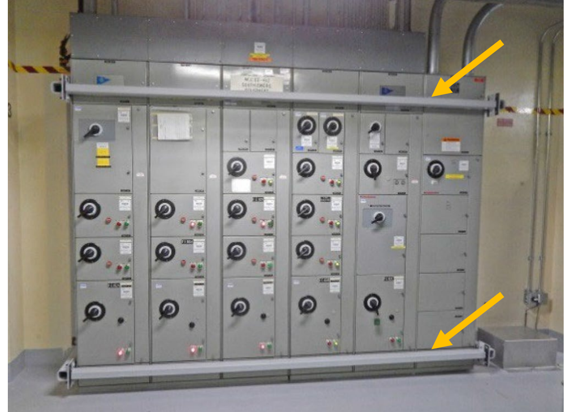
Electrical equipment before (left) and after adding bracing (right) to resist Performance Category 3 earthquakes.
