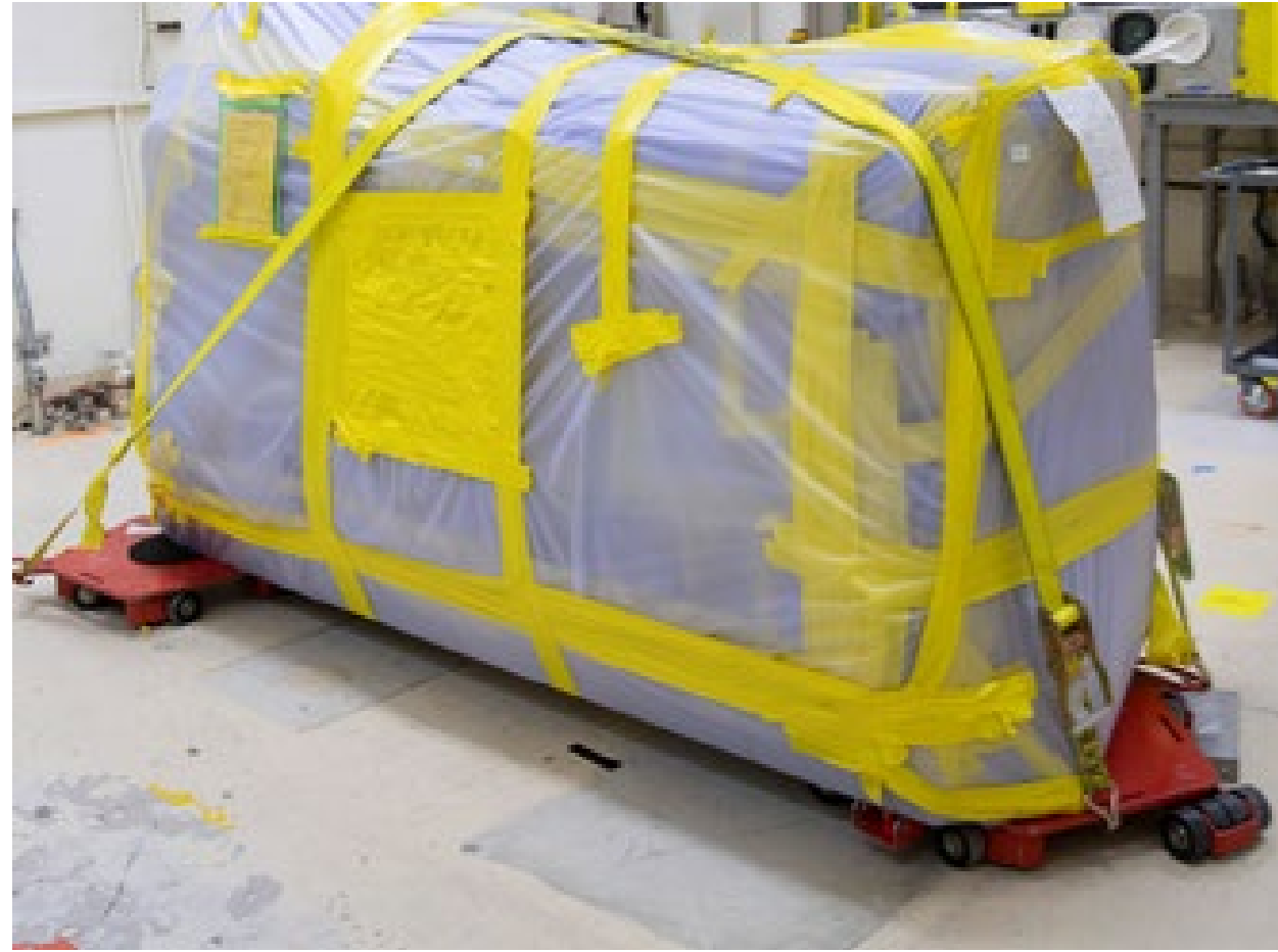
Contaminated equipment wrapped for removal.
