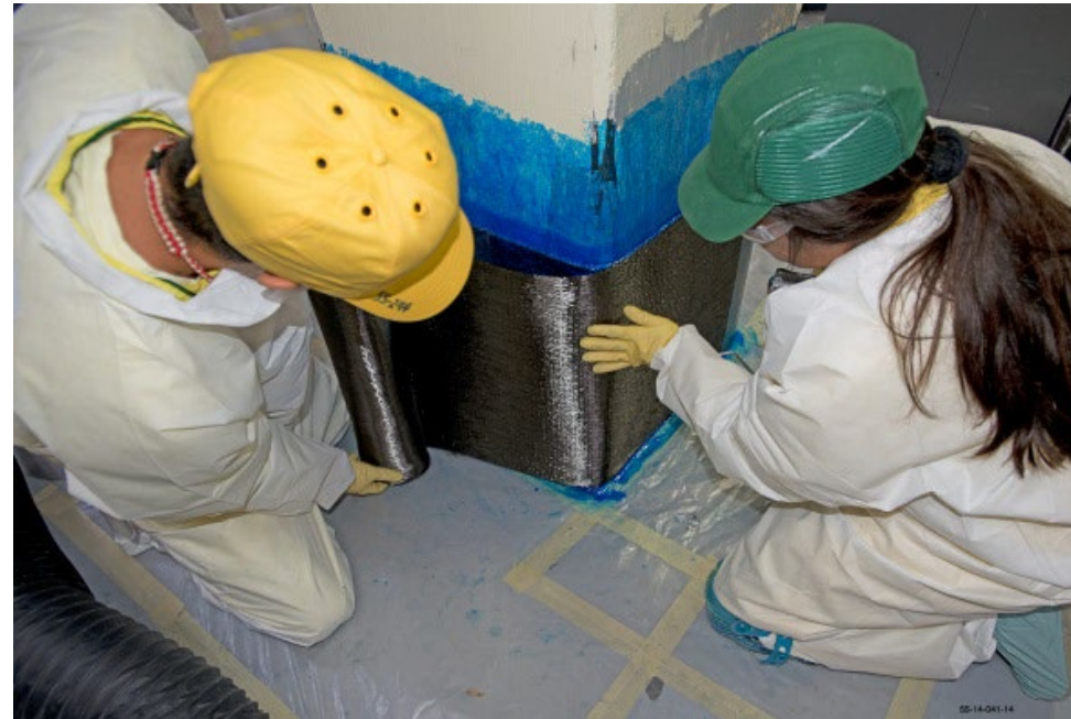
Workers reinforcing structural members. Testing column capitals.
