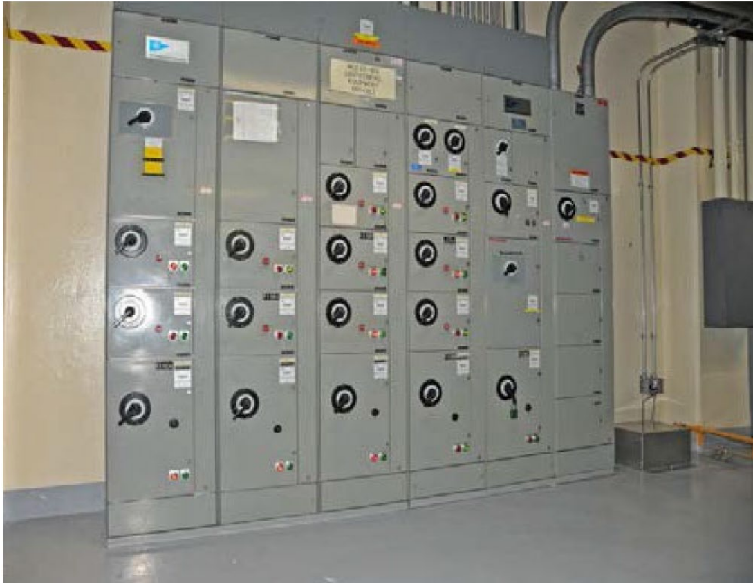
Electrical equipment before (left) and after adding bracing (right) to resist Performance Category 3 earthquakes.
