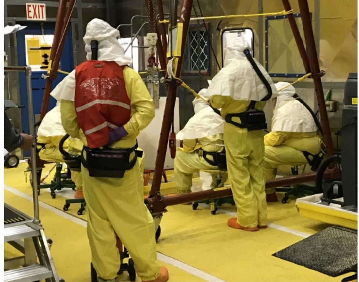
Drill and drain operations.
