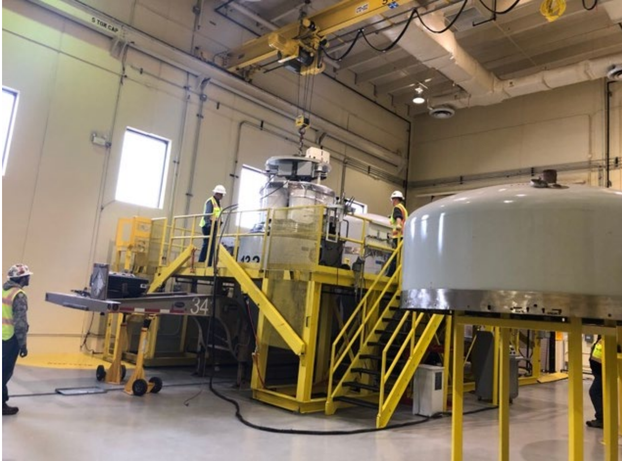
Triad's RANT Shipping Facility.
