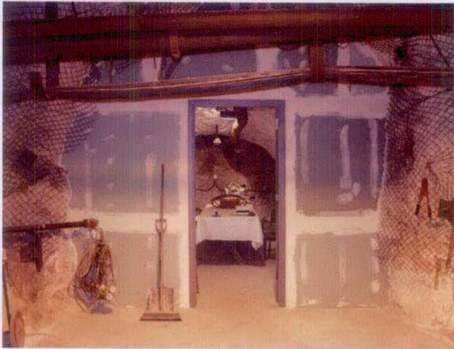
Figure 5-5. Refuge chamber entrance.
