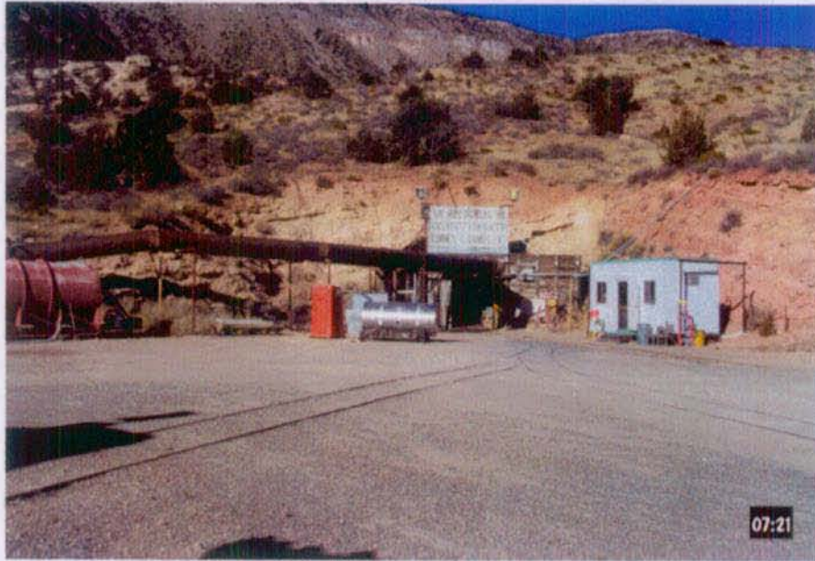
Figure 2-1. U12g Tunnel portal entrance.
