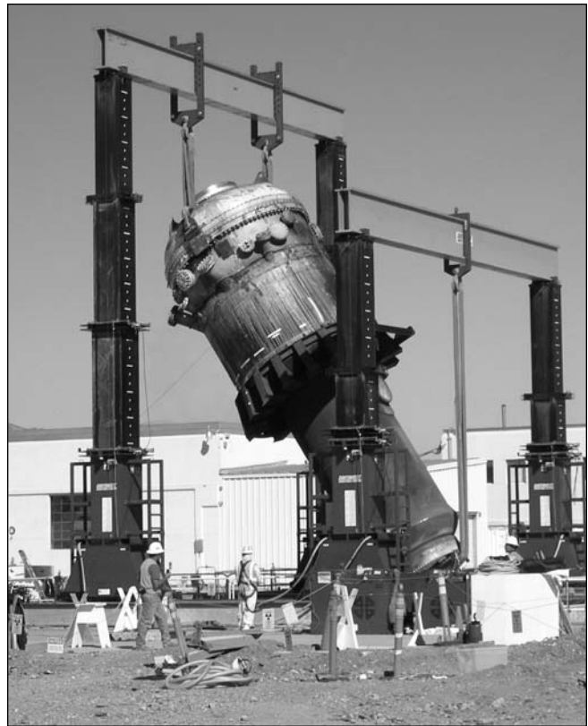
Engineering Test Reactor Removal
