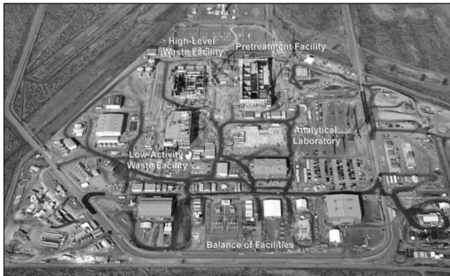
WTP construction progress, October 2006 for comparison to photograph from October 2007 below
