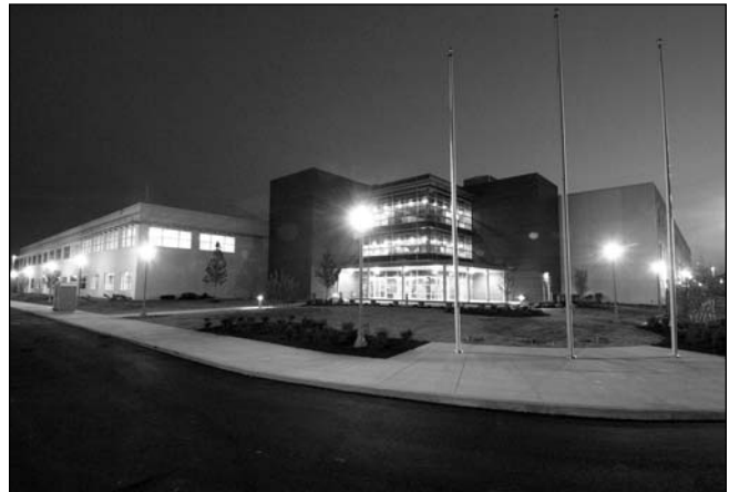
The newly constructed Jack Case Center at Y-12 houses approximately 1200 employees some of whom were previously stationed in Manhattan Project era facilities
