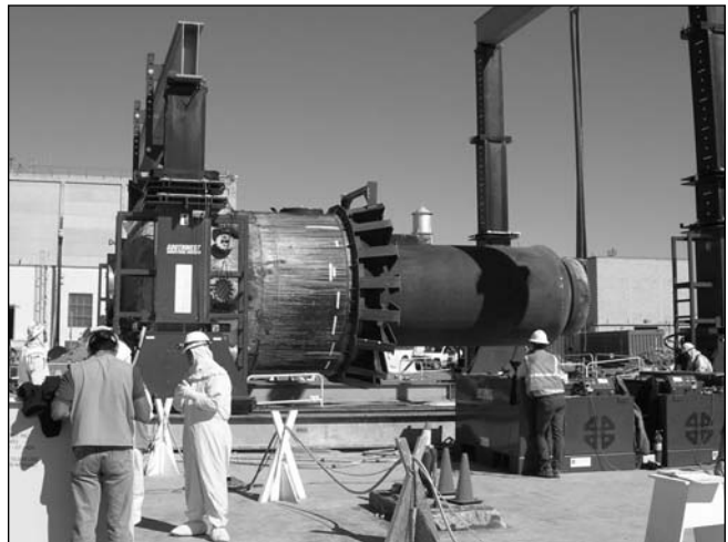
Engineering Test Reactor Removal
