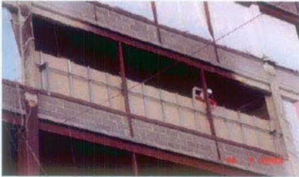
Figure 4 Cardington Facility Test Interior Columns
