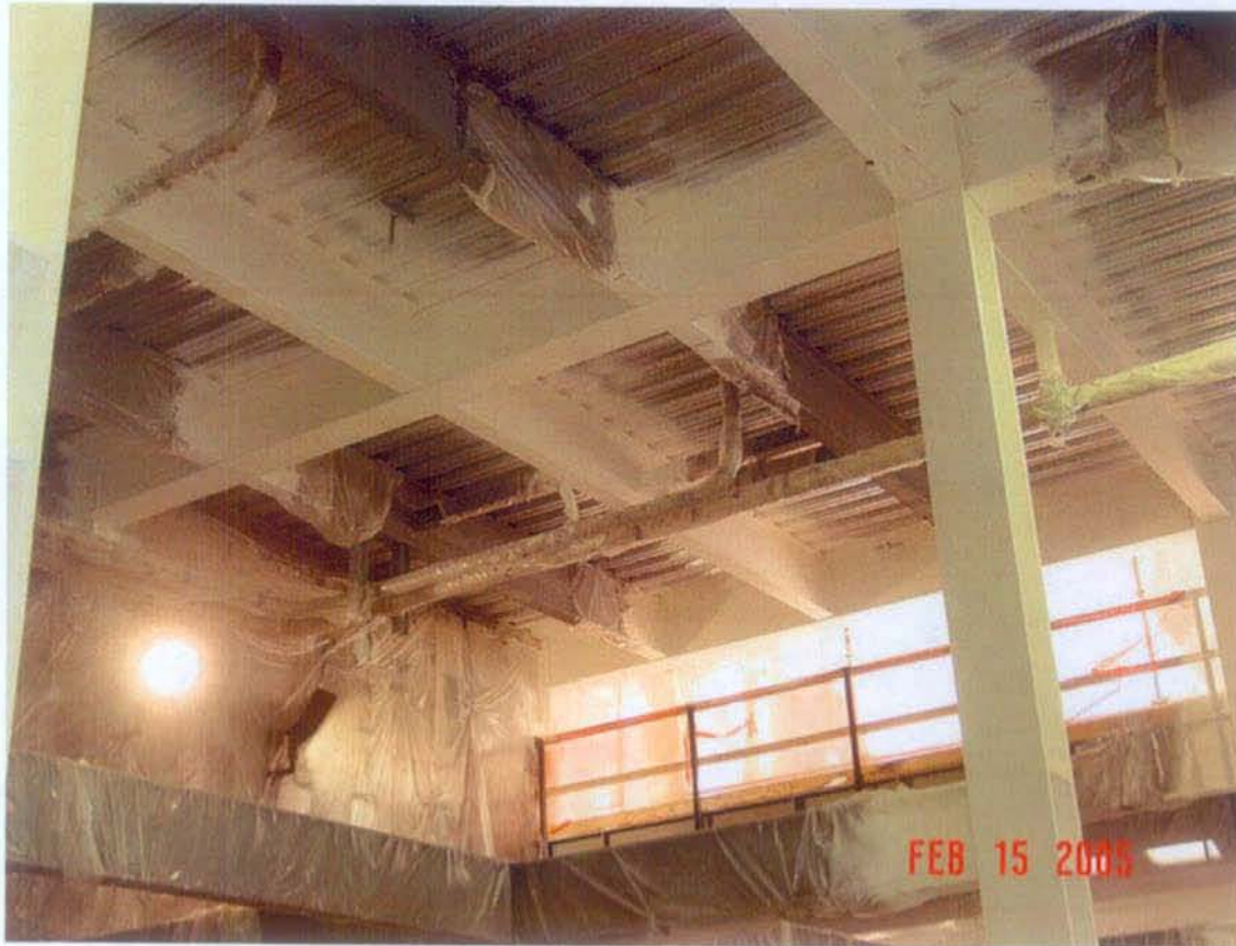
Figure 7 Photograph of LAW Showing FP and NFP Members
