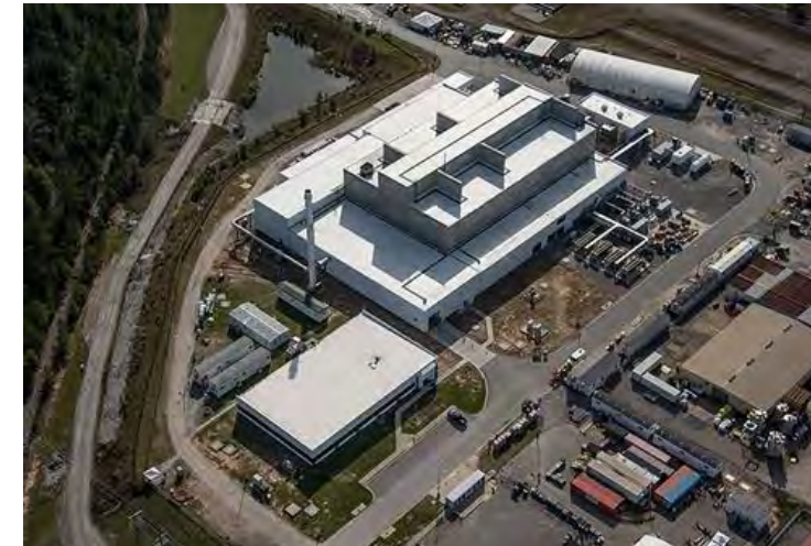
Salt Waste Processing Facility
