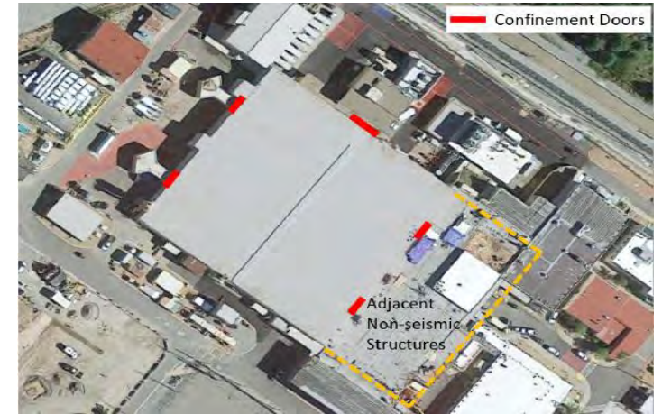
Doors in Passive Confinement for Plutonium Facility at Los Alamos
