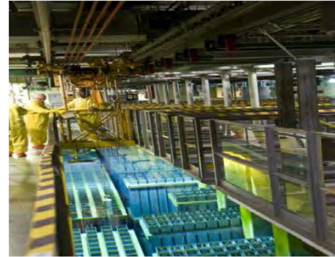
L-Area Spent Fuel Basin
