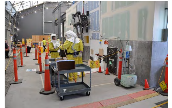
Hanford Site Building 324 High Contamination Area Training
