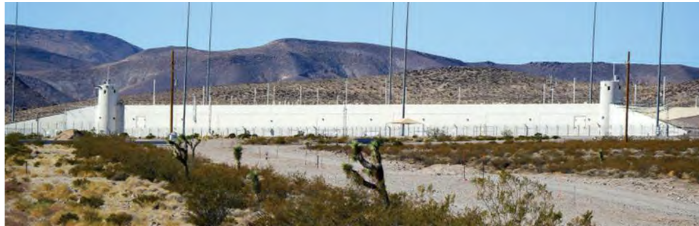
Device Assembly Facility
