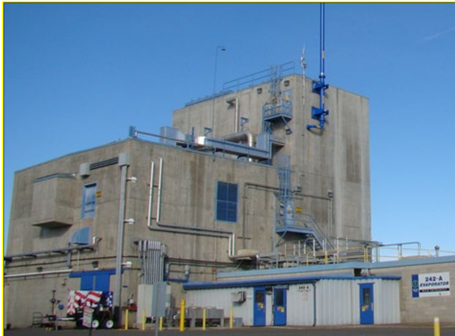
Figure 10. 242-A Evaporator Facility at the Hanford Site
