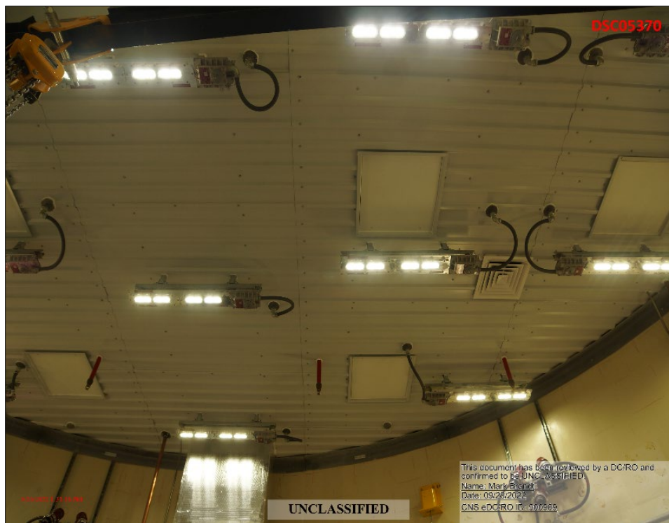
Figure 2. Upgraded False Ceiling within a Nuclear Explosive Cell
