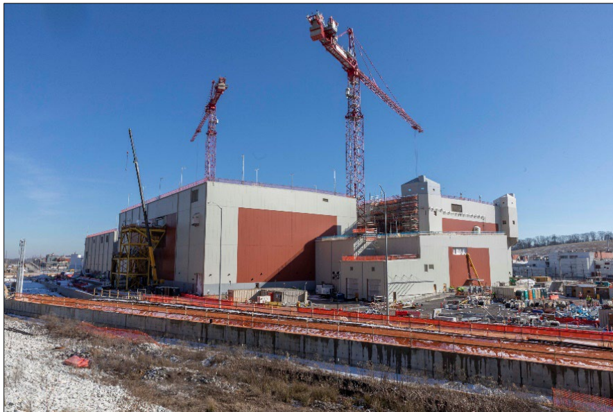
Figure 21. Uranium Processing Facility Construction in 2023
