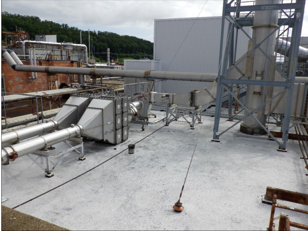
Figure 24. Y-12 Building 9215 Roof Remediation
