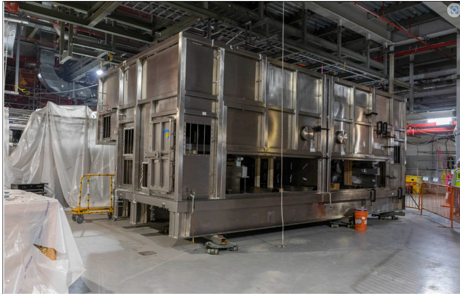
Figure 22. Main Process Building Batch Makeup Staging Enclosure Installation
