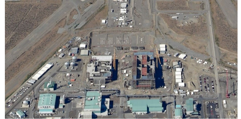
Waste Treatment Plant, Hanford
