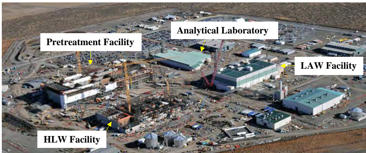
Figure 1. An aerial photograph of the WTP construction site. WTP is composed of four major nuclear facilities: HLW, Pretreatment, Low-Activity Waste (LAW), and Analytical Laboratory. Balance of Facilities provides utilities and support in surrounding non-nuclear structures.
