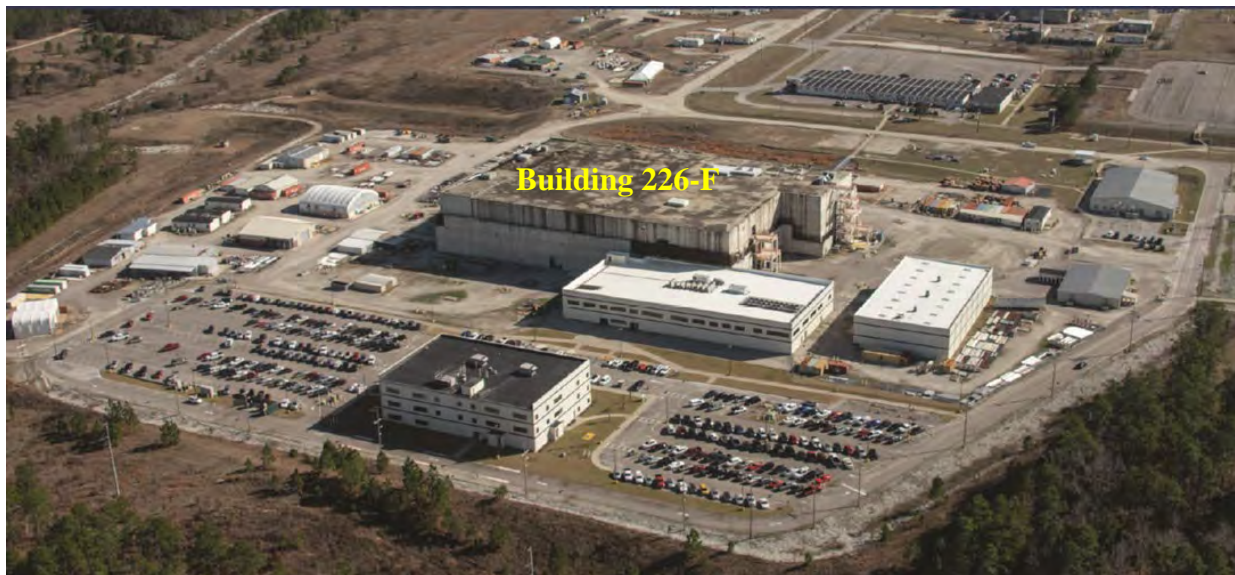
Figure 1. An aerial photograph of the existing structures at the SRPPF site.
