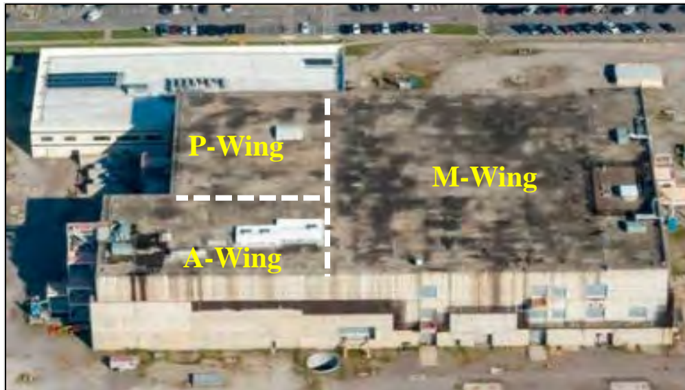
Figure 2. The three wings of Building 226-F at the Savannah River Site. A-Wing and P-Wing have non-safety recirculation ventilation systems and will house workers following an accident.
