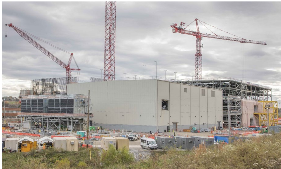
Mechanical and Electrical Building
