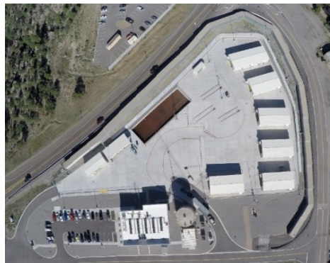
Figure 1. Aerial View of TWF
