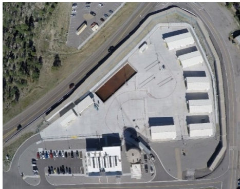
Figure 1. Aerial View of TWF
