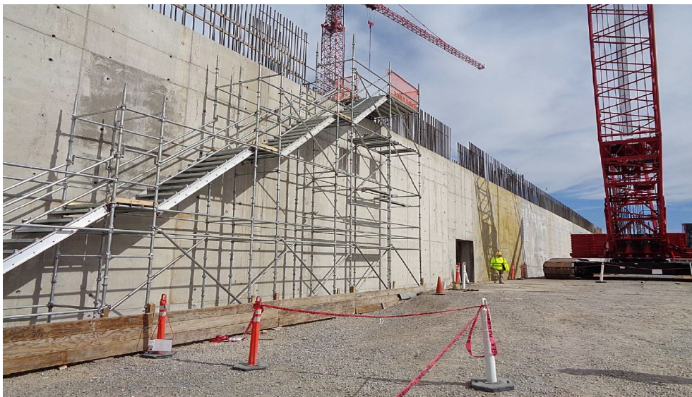
UPF Main Processing Building Construction
