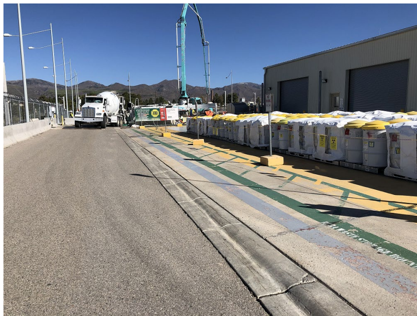
Transuranic Waste Storage Outside of the Plutonium Facility
