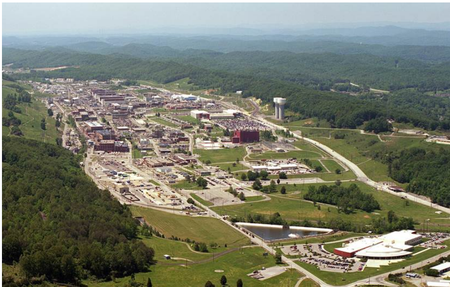
Y-12 National Security Complex
