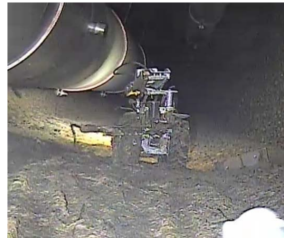
Crawler Inspection of SRS H-Canyon Exhaust Tunnel
