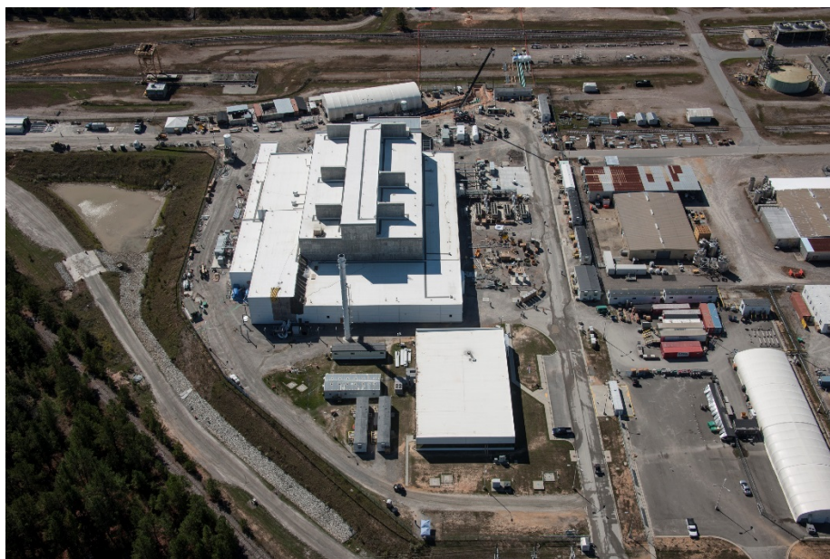
Salt Waste Processing Facility at the Savannah River Site
