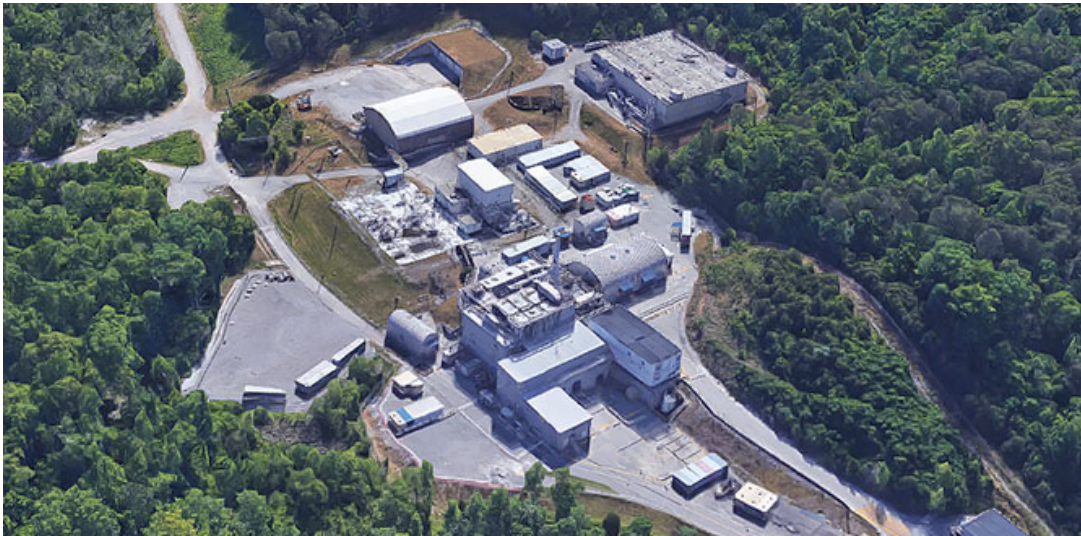
Transuranic Waste Processing Center at ORNL
