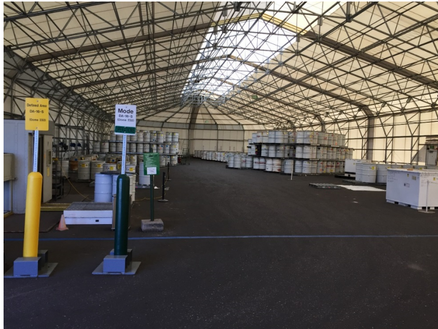
Waste Drum Storage at LANL Area G Dome
