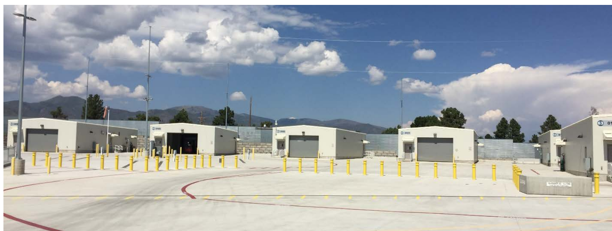
Figure 1 – Completed Transuranic Waste Facility
