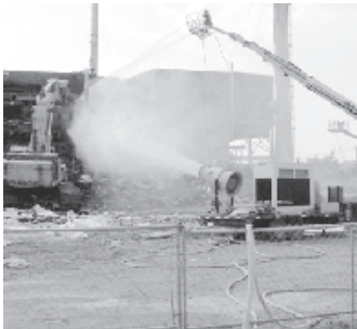
Demolition of the R/SW building at the Miamisburg Closure Project.
