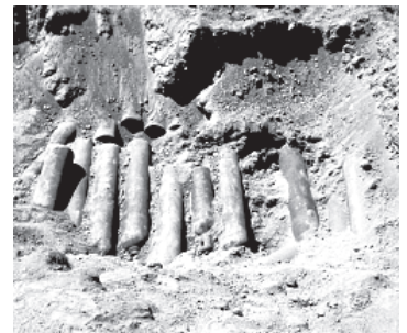
Deactivation, Decommissioning and Demolition of cylinders at the Idaho Nuclear Technology and Engineering Center.
