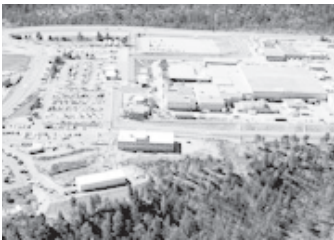
Las Alamos National Laboratory Plutonium Facility.
