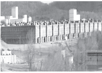
Side view of the K-25 Building at the East Tennessee Technology Park in Oak Ridge, Tennessee, that is currently undergoing decontamination and decommissioning.
