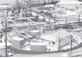
An aerial view of the H Tank Farm at the Savannah River Site.
