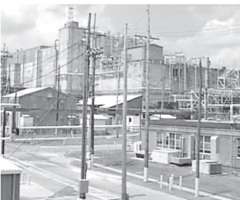
F Area Complex at the Savannah River Site.
