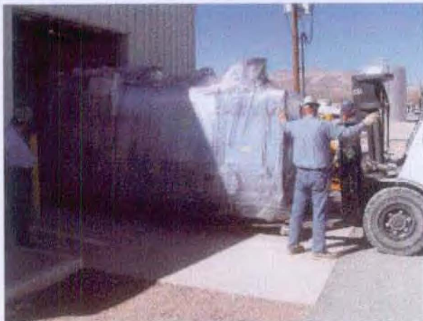
Glovebox Removed. The Glovebox Previously Used in the Area 5 Visual Examination and Repackaging Building to Characterize the TRU Waste Was Removed and Disposed of On Site
