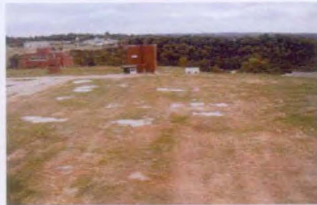
After Photograph of MCP From Operational Support West Building
