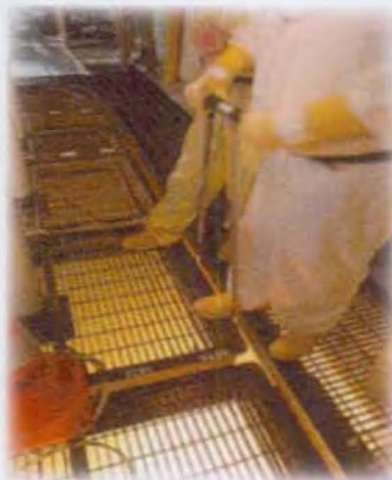
Consolidated Radioactive Sludge (an Estimated 55 Cubic Yards) Vacuumed from the Floors of Hanford's K East Basin. Began Transferring the Sludge Out of the Basin in Preparation For Draining and Removing the Leak-Prone Pool
