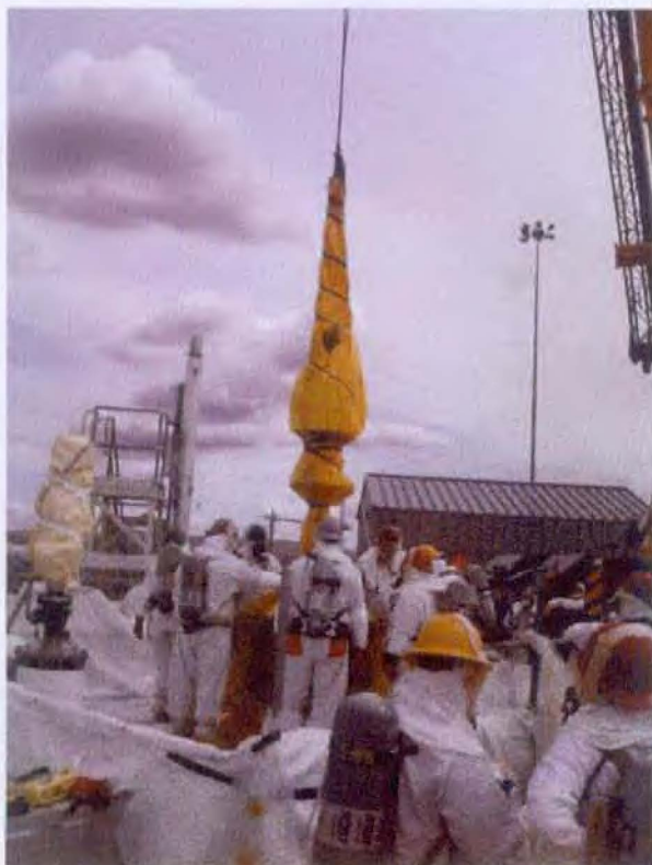
Removing a Failed Sluicer at Tank C-103
