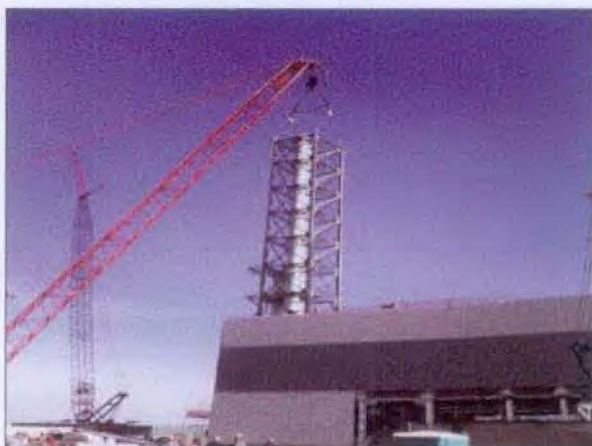
Setting of Low Activity Waste Facility Stack
