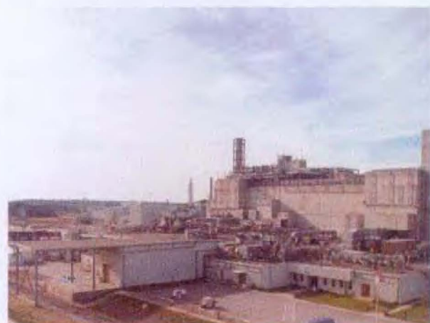
Defense Waste Processing Facility
