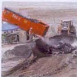
Contaminated Soil and Other Material from Hanford's River Corridor Is Being Disposed of in the Environmental Restoration Disposal Facility. Water Is Being Applied for Dust Control
