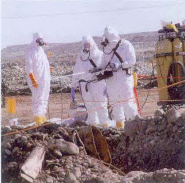
Drums Unearthed from a Burial Ground Near the Columbia River in Hanford's Reactor Areas Are Surveyed for Contamination
