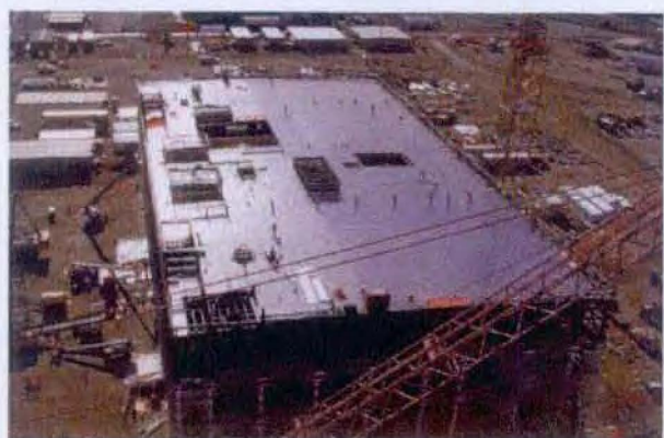
Prepping Roof on Low Activity Waste Facility
