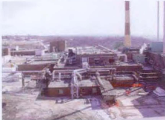
Before Photograph of MCP From Operational Support West Building
