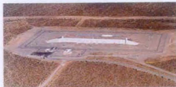
The Device Assembly Facility (DAF) at the NTS Was Used to Support the NNSA Off-Site Recovery Program (OSRP)
