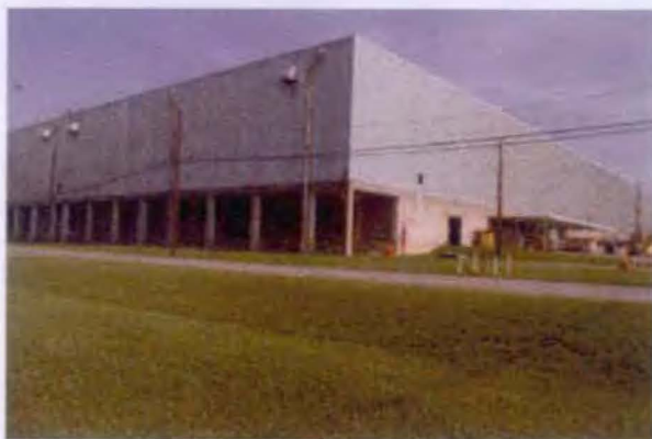
Southeast Corner of the K-29 Building
