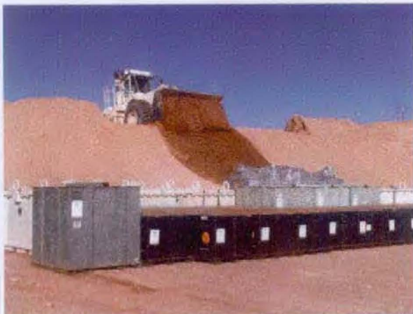
Glovebox Burial. The Low-Level/Mixed Low-Level Waste (LLW/MLLW) Project Facilities Located in Area 5 of NTS Provide Disposal Services for On-Site and Off-Site DOE Generators
