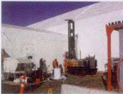
Accelerated Retrieval Project Foundation Stabilization
