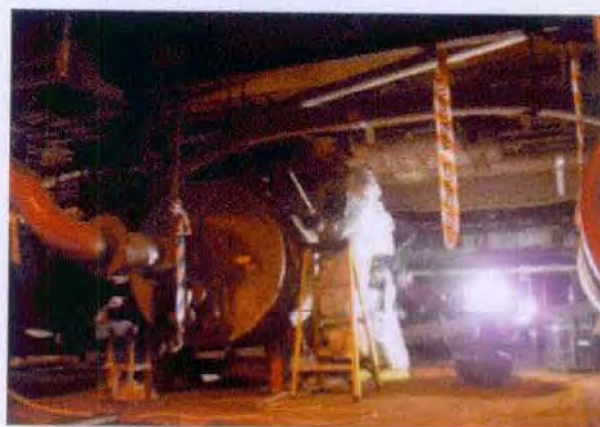
Vent/Purge/Drain Activities in K-25 Building
