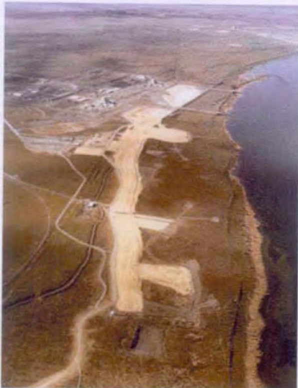
Recently Completed Remediation of the Liquid Waste Trench in Hanford's K Reactor Area. Contaminated Soil From the "Mile Long" Trench Has Been Removed, then Backfilled and Vegetated. It is Adjacent to the Columbia River
