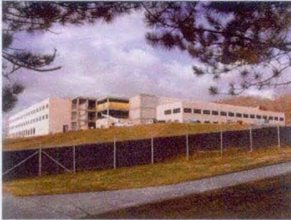
View of the Privately Financed Jack Case Center Under Construction at Y-12
