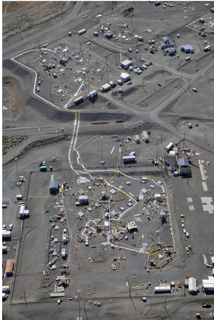
Hanford Tank Farms Aerial View
